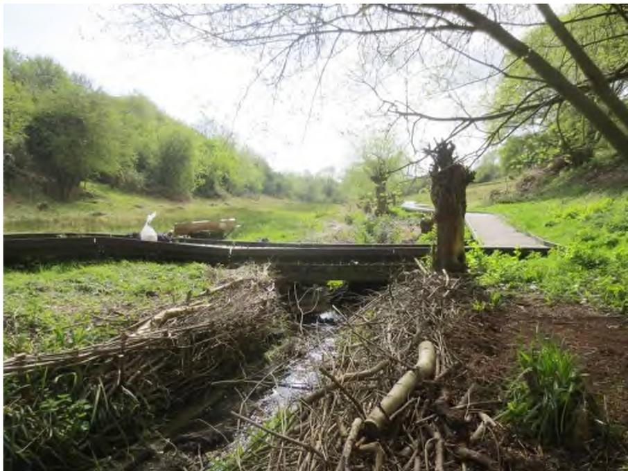
*Near the bridge, bank erosion has been stopped by installation of protective hazel wattle structures by FoLV volunteers.*
