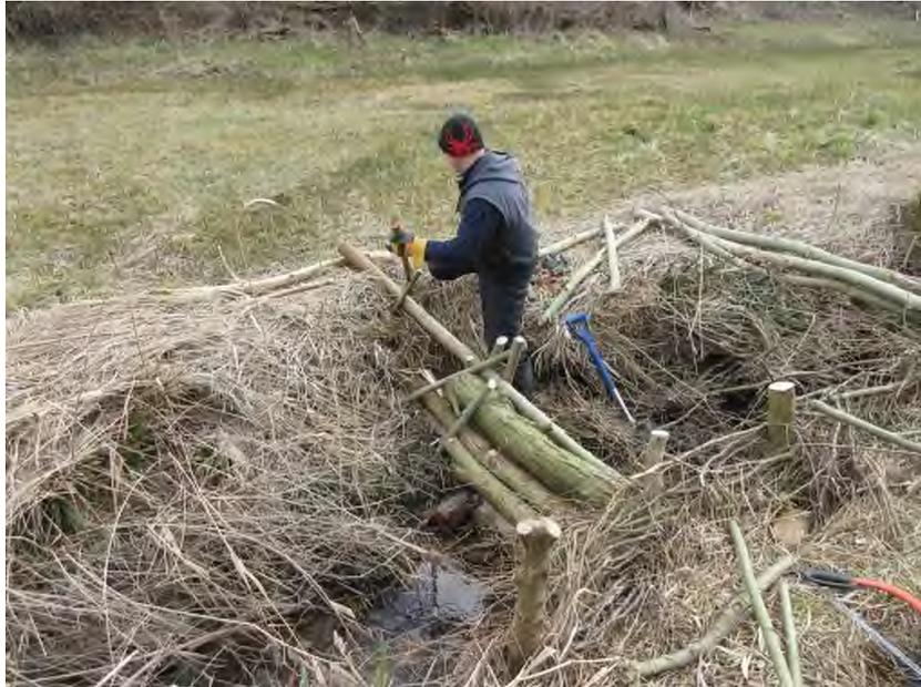
*Leaky log dam installation in the SSSI section 20.03.2018*
