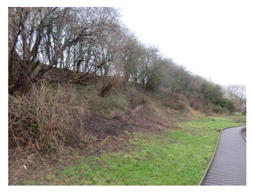
Tipped embankment of made ground (left, slope angle 32 to 42 degrees) to the Warren Crescent site at top left behind the trees. View looking north from the boardwalk through fen in Lye Valley bottom. 13.01.2021 J.A.Webb
